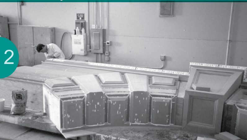
The Flood Building under restoration in 1992
